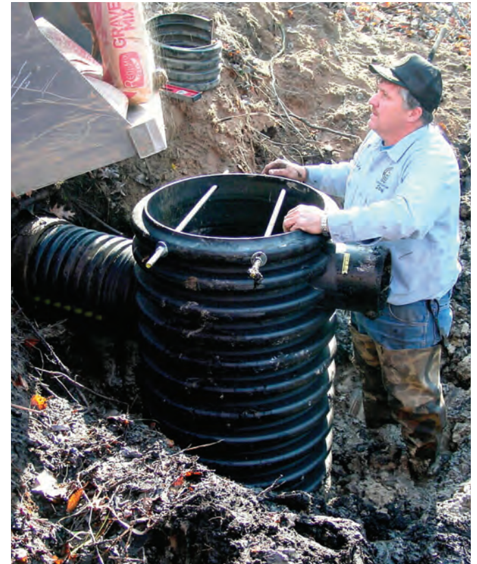
Placing riser on the southwest tributary.
